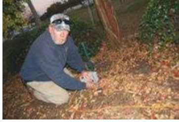
Lake City public works employee Sam Pate checks the power supply to some lights in the city's holiday display Monday. (Staff Photo: Curt Yeomans)
